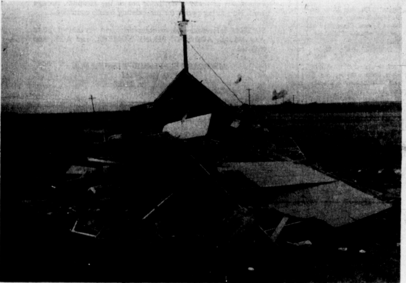
THIS IS WHAT IS LEFT of LaGrone's Liquor Store on Highway 70 after a tornado struck it Thursday.
