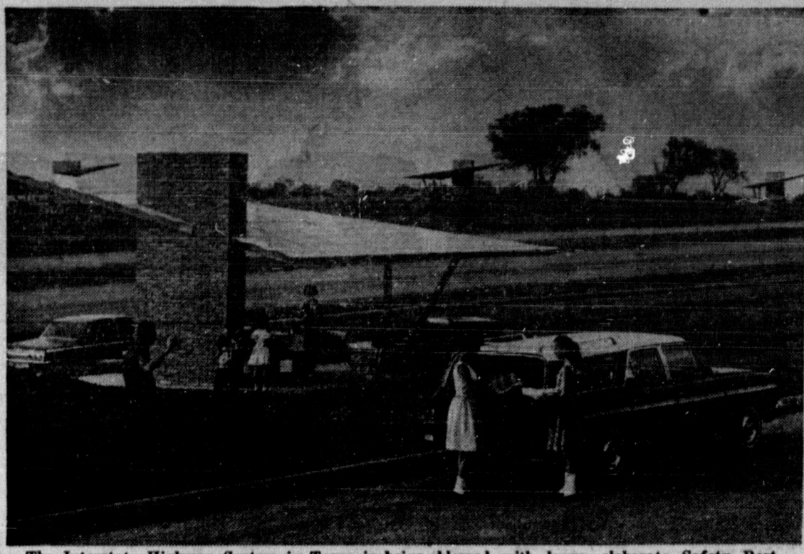
The Interstate Highway System in Texas is being blessed with large, elaborate Safety Rest Areas for the safety and convenience of Texas travelers.
