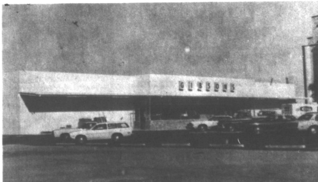
GIBSON DISCOUNT CENTER , Clarendon's newest business, is nearing completion at its location on Highway 287 with plans to be open by next weekend and have a Grand Opening beginning Tuesday, November 25. The 20,000 square foot building will contain a complete food and family center. James Stubblefield is the local manager. The business is owned by Alex Saied, long-time Childress businessman, who operates a large Gibson store there.
