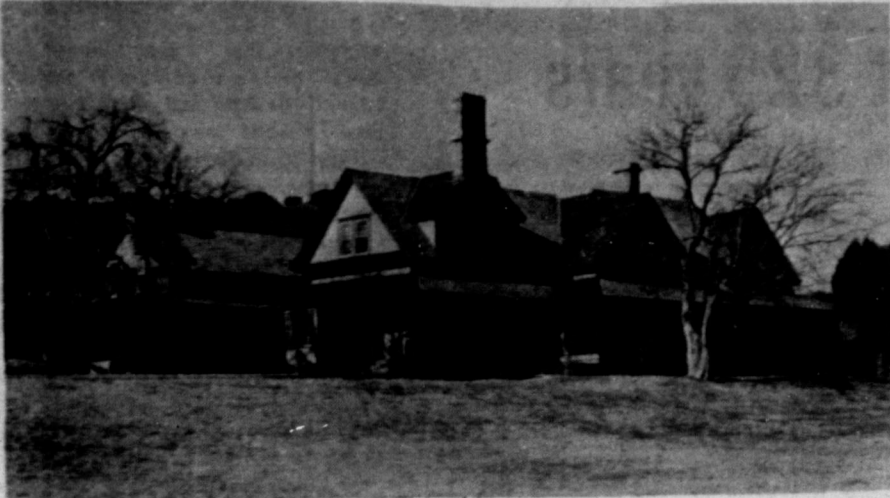
PRESENT JA RANCH HOUSE
