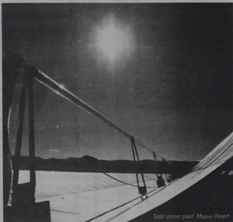
Solar power plant, Mojave Desert
