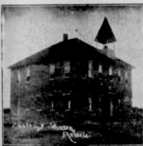
HOPE SCHOOL BUILDING.
