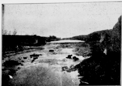
Dam on the PECOS RIVER.
