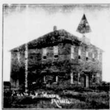
Schoolbuilding at Hope, New Mexico made of Artificial Stone manufactured and put up by I R Daniel
