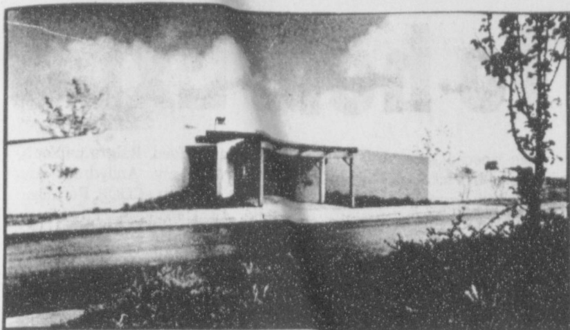
The Ronald McDonald House of Amarillo, front entryway.
