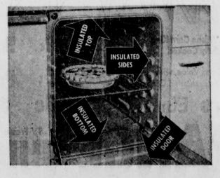
An electric range oven is insulated all around, including the bottom, to keep heat inside where it belongs. This is possible because the electric oven, being flameless, does not require a flow of air into and out of it to support combustion. Result: your kitchen stays cooler when you are baking or roasting.
