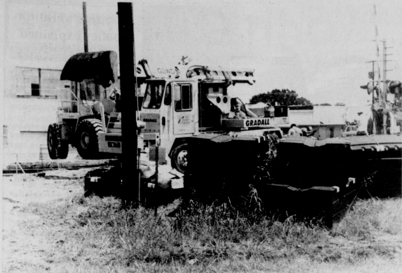
IMPROVING A BAD SITUATION - Burlington Railroad crews began a long-awaited project Monday, to replace the old and rough wooden cross-ties on Yosemite, with rubberized material, shown stacked in the lower right. Work reportedly is to be completed today.
