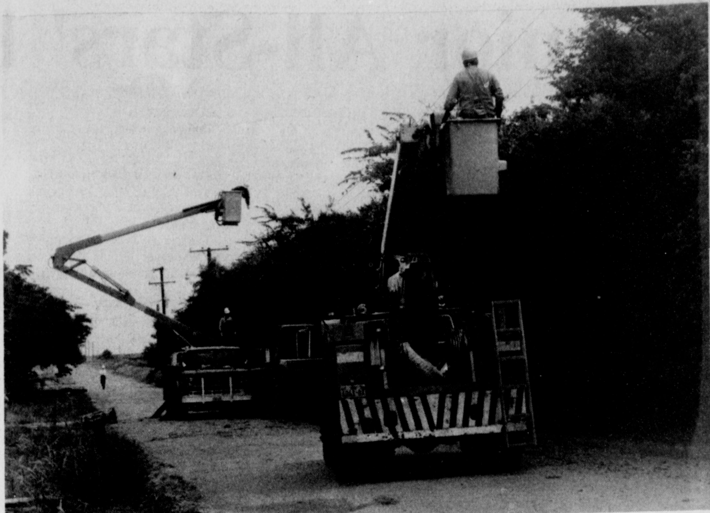
ELECTRICITY SERVICE RESTORED - TU Electric crews are shown making a temporary repair of broken lines Monday morning on Bell Road. The outage affected most of the east and south-east part of the city, and some was not restored until 3 p.m. Telephone and cable service was also discontinued to many residents. A TU Electric spokesman said Freddie Daume would be billed for the cost of repairs. Daume admitted he broke the lines when his plow was snagged.
