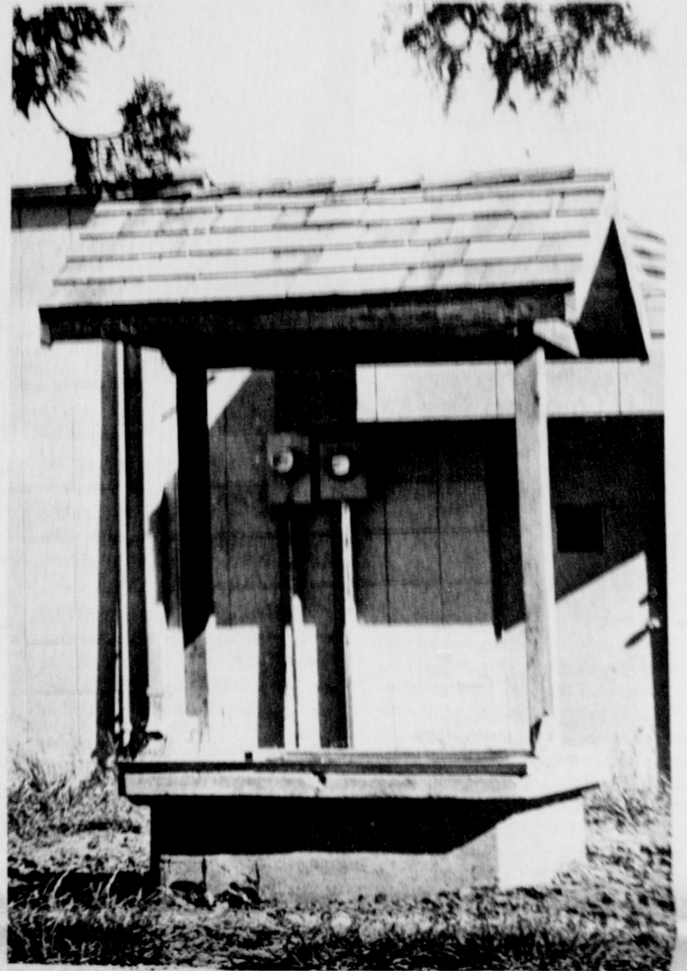
WELL MADE ATTRACTIVE - An old well, located on the east side of city hall, was made more attractive recently when workers built a cover over it. No records are available at city hall on the well's history, and anyone knowing its background is asked to contact the Leader.
