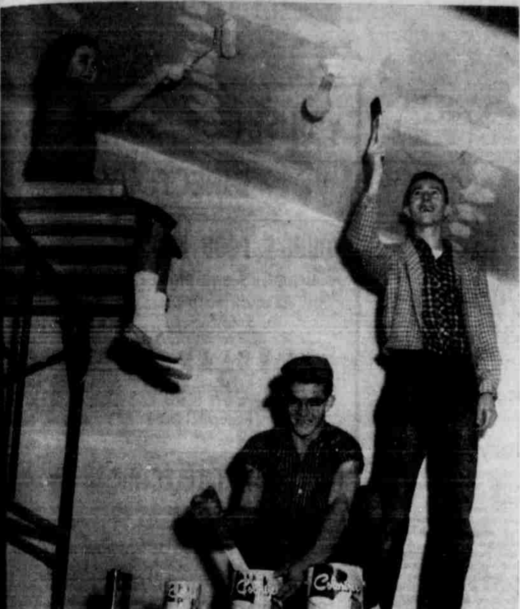
IT ISN'T EXACTLY WORK These three 4-H Club members are among the volunteer workers helping finish the new 4-H building on the south side of the City-County Park. Seated on the scaffold is Judy McCampbell, 11, daughter of Mr. and Mrs. J. D. McCampbell. Donald Young, son of Mr. and Mrs. Alvin Young, mixes paint, while Don Richardson, son of Floy Richardson, applies the brush. (Staff Photo.)
