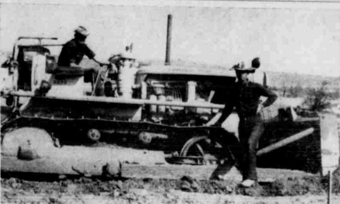
THEIR JOB IS BUILDING TANKS —These two employees of Texas Dirt Contractors are shown on the Tom Sims Ranch, north of Post, where they are excavating for a ranch pond. At the right is Nathan Little, who is in charge of the dirt-moving outfit, and on the scraper-equipped "cat" is Leland King. Not quite visible in the rear of the picture is Keith Adams, who is working on a bulldozer.—(Staff Photo.)
