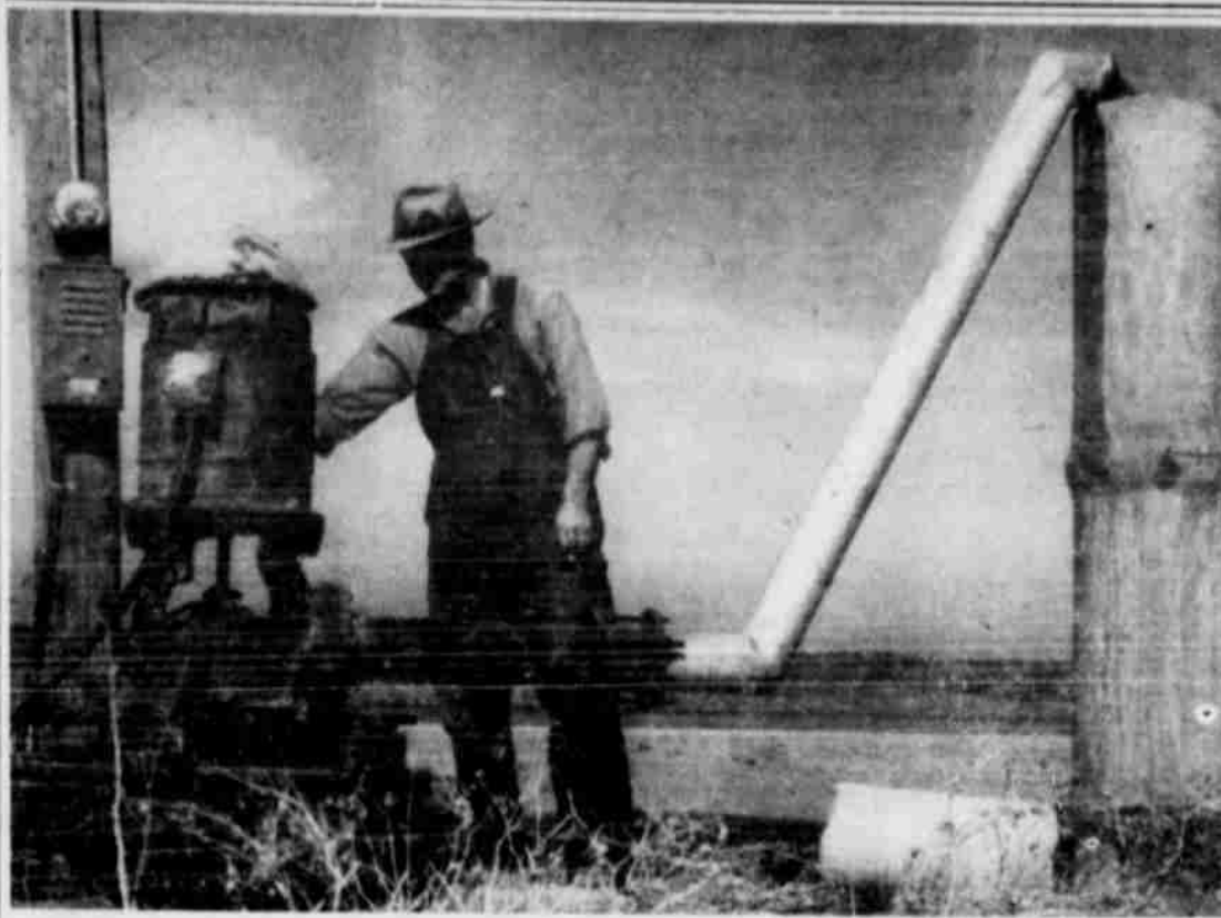
CONCRETE PIPE STARTS HERE—Shown here is one of the two irrigation wells on the Will Teaff farm from which water is pumped through 1,900 feet of concrete pipeline installed early last year. Teaff and his son, Howard, shown in the picture, are firm believers in the value of concrete pipe for irrigation purposes.
