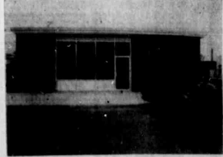
NEW CABINET SHOP Formal opening of the Ben Owen Cabinet Shop at 318 East Main is to be held Saturday, April 28, with three prizes to be given visitors. The new all-steel building is 36 by 75 feet.—(Staff Photo)
