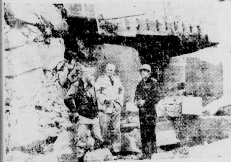
Three American naval officers stand amid the wreckage of the arsenal at Cherbourg, graphic testimony to the efficiency of German demolition squads. Left to right are Commodore William A. Sullivan, port salvage expert; Rear Adm. John Wilkes; and Rear Adm. Alan Kirk, commander of U. S. naval task forces in French waters.
