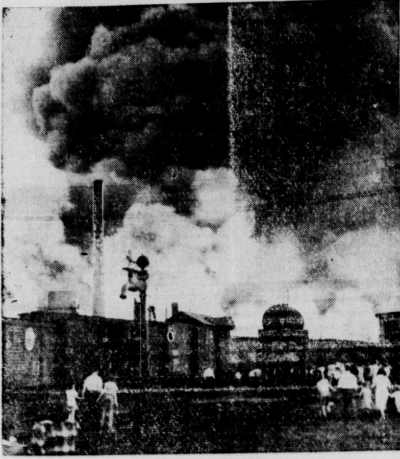
Photo made from Boston & Maine railroad freight yard in Charlestown, Mass., shows clouds of smoke billowing over freight cars. All Boston police and firemen on duty or off were called to the scene, as were coastguardsmen from the navy yard. Apparatus from six adjacent cities aided. There were five casualties, and the loss was estimated at $750,000.
