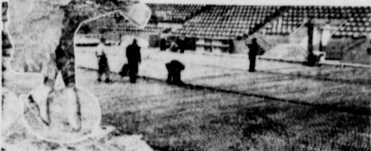
STAGE FOR EACH SHOW, carried about the nation in trailers powered by International track-tractors, is 9,000 square feet of piping. Brine is circulated through the piping which is then covered with water. Freezing action quickly creates smooth skating surface.
