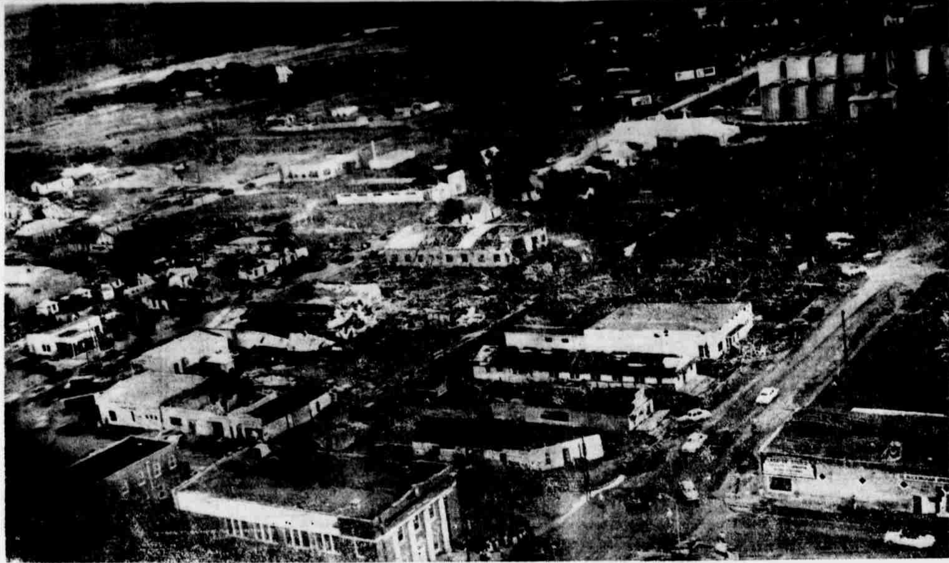
Part of the business section of Olney laid waste by the destructive tornado which struck that city Friday afternoon in which two persons were killed and several injured is shown in the above aerial photograph made by a photographer of the Fort Worth Star Telegram.
