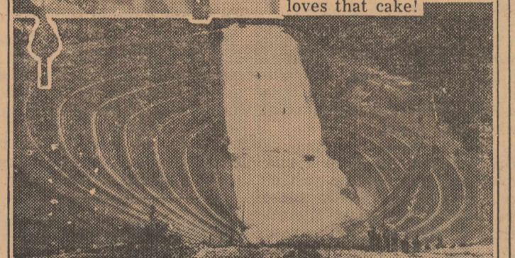
GREEK STYLE amphitheater to seat 60,000 for ski jumps is being built at Innsbruck, Austria, for 1964 winter Olympics. Here they pack in some imported snow for an inter-city jumping tournament.
