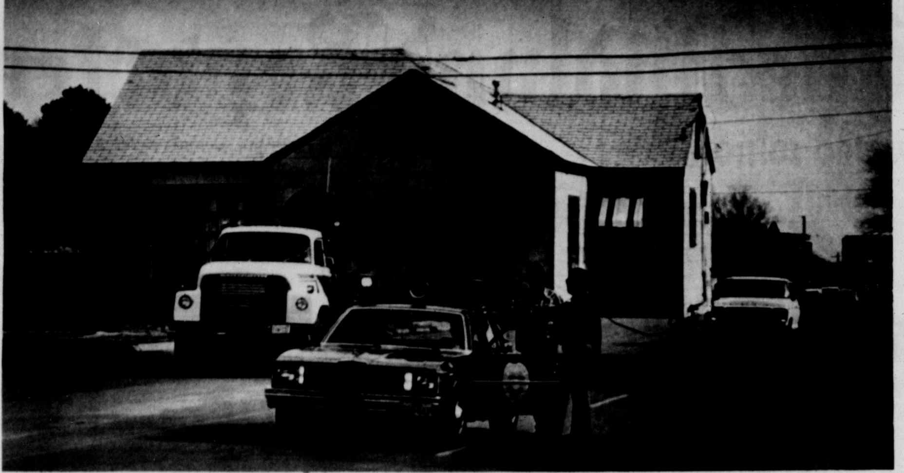
Workmen and a police escort pause as they wait for electrical lines to be raised near the intersection of Wall Avenue and G Street shortly before noon Monday. The home finally made it to its destination in the 4000 block of Tanner later in the day. (Staff Photo by Brian Hendershot)
