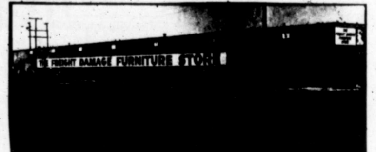
2900 WEST FRONT ST. THE BIG PURPLE BUILDING
