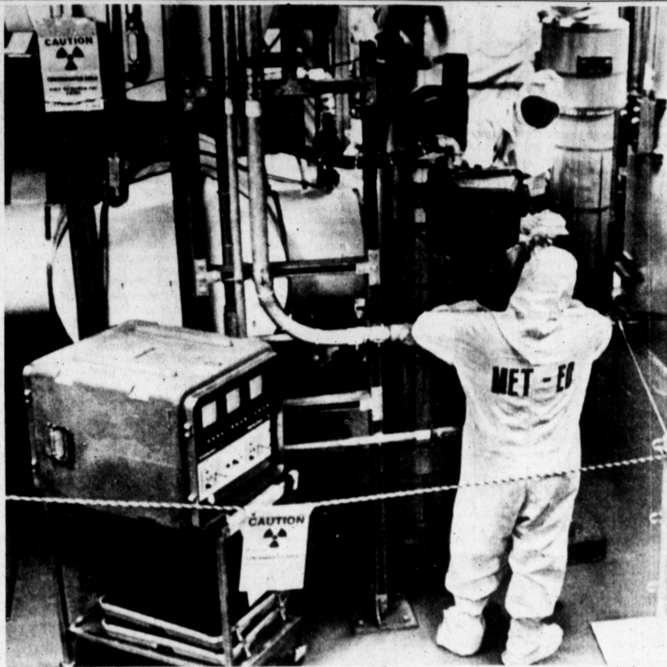
Two Three Mile Island technicians wearing protective clothing decontaminate a heat exchange system in the Unit 2 auxiliary building next to the nuclear power plant near Middletown, Pa. News-
