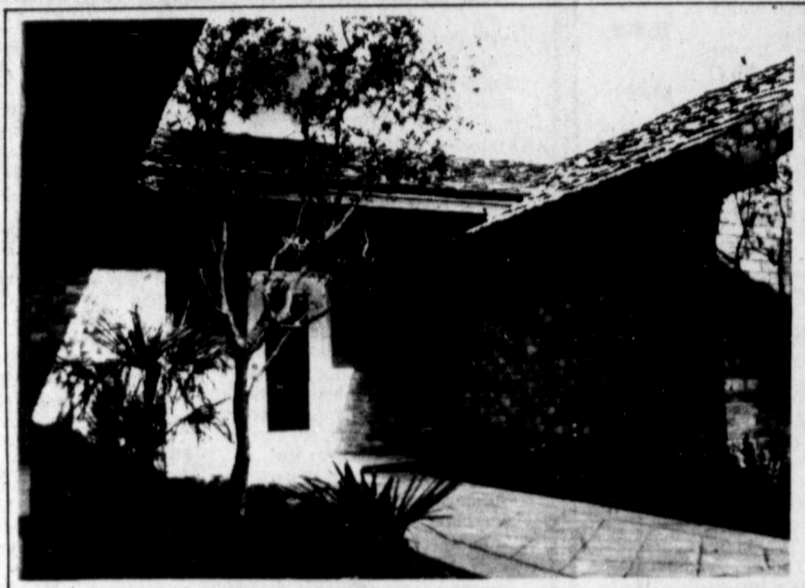
This lovely patio home at 4805-1 Spring Meadow Lane in Meadowpark is one of 12 now nearing completion. Three others now complete will also be open Saturday and Sunday. The builders, and representatives of Citizens Savings, will be available to answer your questions.
