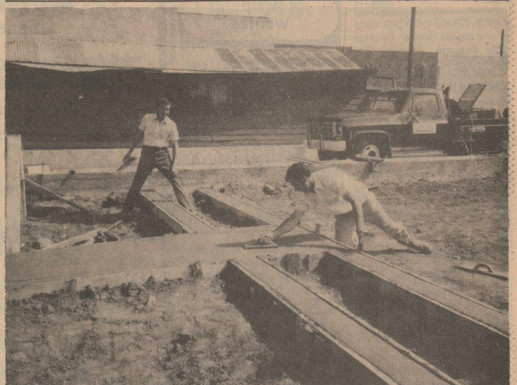
DONATING TIME and labor last week on the Knox City Downtown Parking Lot project were Glen Rumley and Greg Kuehler, pictured here as they finish smoothing the cement last Thursday morning. David Counts, project chairman, expressed thanks to these men for assisting and said that the other area would be hot-topped soon. (Picture courtesy of David Counts)
