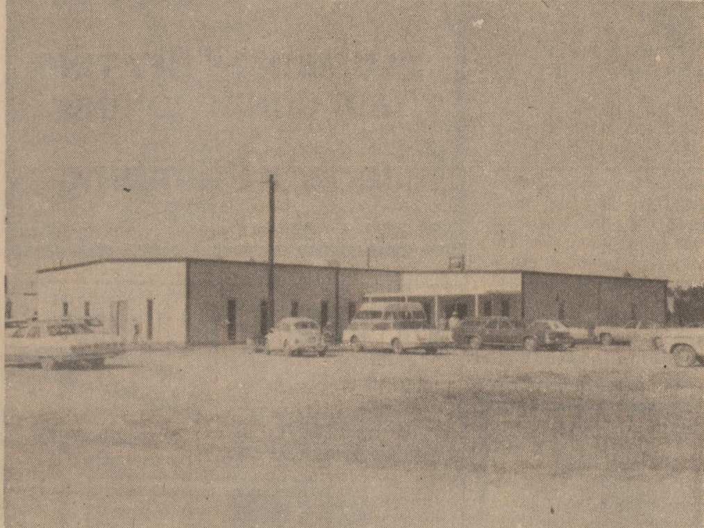
THE SPACIOUS BENJAMIN MEMORIAL CENTER was dedicated during ceremonies Saturday afternoon. Plans for the building began four years ago and Jim Bob Bisbee, president of the Benjamin Ex-Student Association was lauded by the exes for his 'dream, fortitude, and drive' making it a reality.
