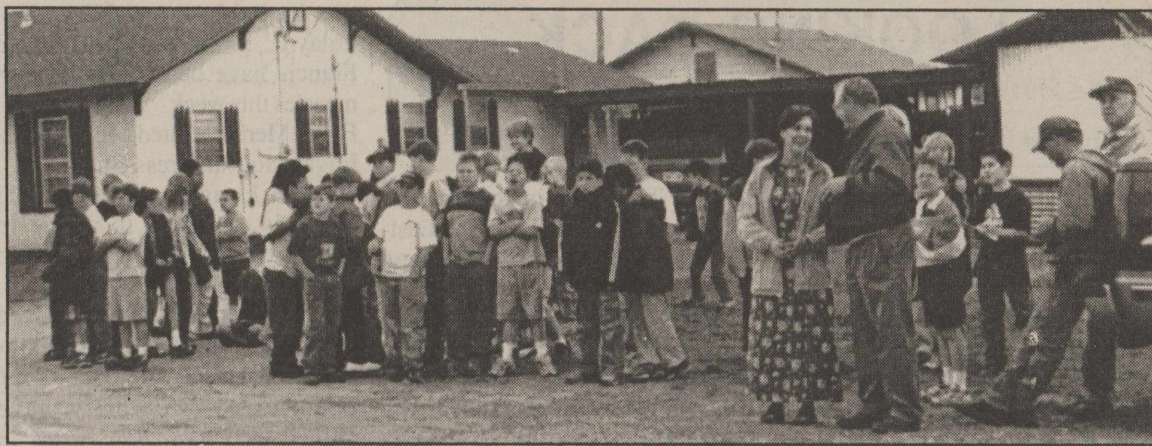
Silverton School students were allowed to watch the raising of the new water tower on Tuesday morning of last week. The operator of the giant crane was very good at his job, and those who helped guide the tank into place seemed fearless as they worked at the top of the base.
