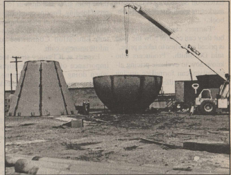
Silverton's new water tower is being constructed and will be going up in a few days, weather permitting. The tower cost $340,000.00, and of this amount, the City of Silverton received a grant for $250,000.00 to reduce the cost of the project. The new water storage facility will be in the shape of a "golf ball on a tee." Briscoe County News Photo
