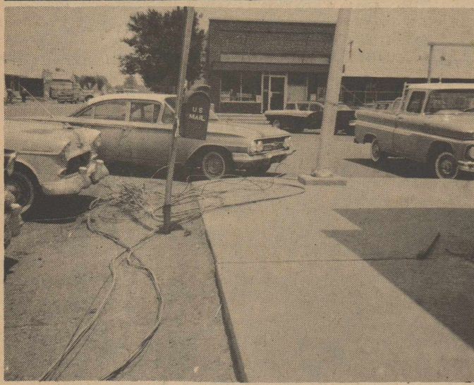
LINES DOWN --Shown above are telephone lines downed in Hart Sunday night by an oil rig passing through. Damage was estimated at $4,000 to $6,000.
