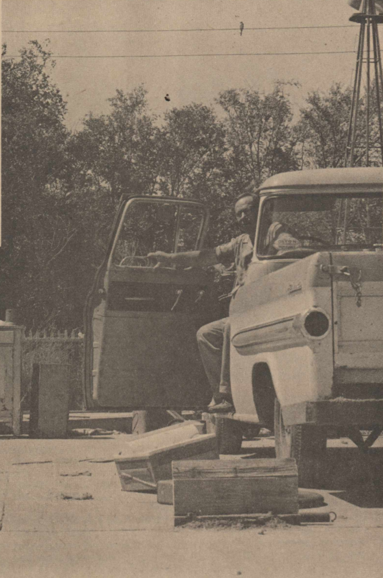
of the garage that were not moved by the storm. In set above is the garage roof which was thrown over a fence at the rear of the home.
