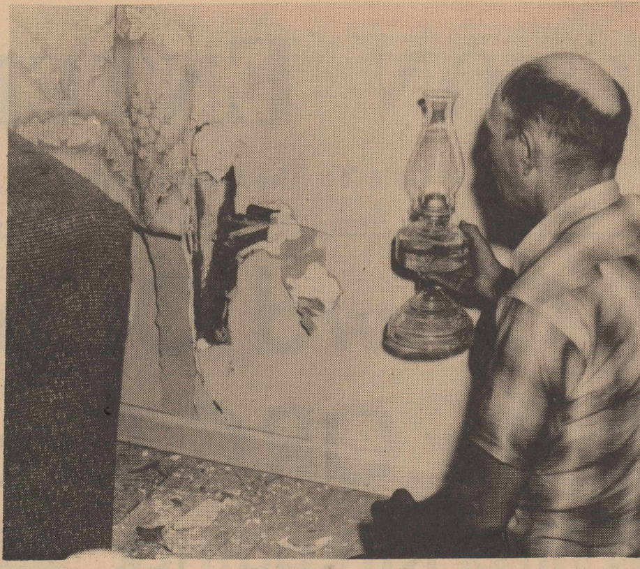
INSIDE THE PIGG HOME, Henry Pigg shines a lantern at the place where a landing gear blasted this hole in the wall, shoving the couch outward. "I thought the house exploded", Pigg said.
