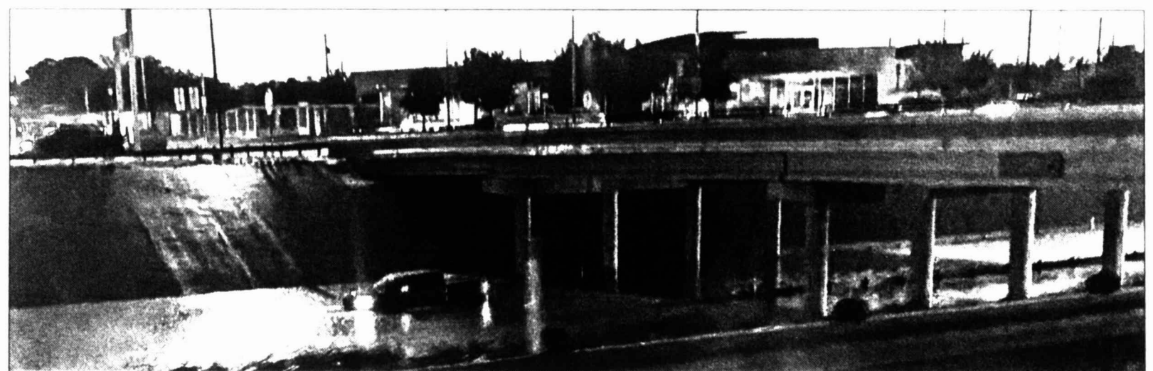
Underpass floods ... Several vehicles were stranded and traffic was halted in Tahoka on US 87 during heavy rainfall Sunday evening, after two underpasses in Tahoka flooded. About 25 stranded travelers were shuttled to safety to the First Baptist Church fellowship hall, for the duration of the storm. (PHOTO by Jeremy Antu)
