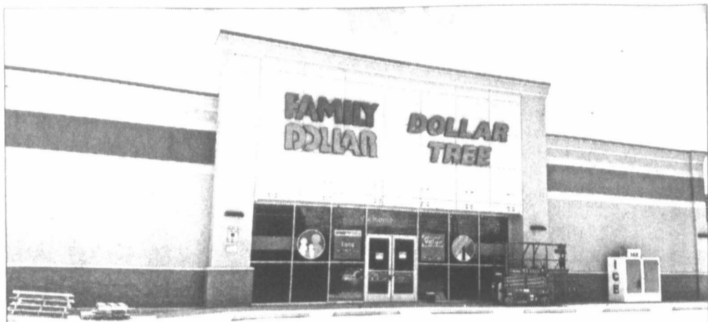
Progress ... Tahoka's new Family Dollar/Dollar Tree store is nearing completion, with work appearing completed on the outside of the building in the 1700 block of Lockwood, and progressing on the interior of the building with shelving and furnishings. No official word has been received as to when the new store will open. (LCN PHOTO)
