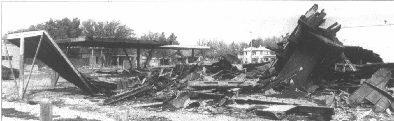
Going to rebuild ... This week the charred remains of the Dixie Dog Drive-In in Tahoka, destroyed in a fire last October, were being demolished. Owner Mercy Tejada says the family is going to rebuild a new Dixie Dog in the same location on Main Street. (LCN PHOTO by Pam Elrod)
