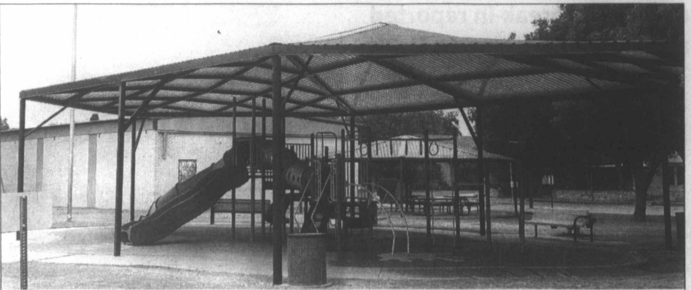
New awning ... The Tahoka Economic Development Corporation (TEDC) had a new metal awning placed over the playground at the Tahoka Minipark, to replace the damaged canvass awning that previously covered the area. The new awning, at a cost of $7,000, covers a larger area than the previous awning. (LCN PHOTO)
