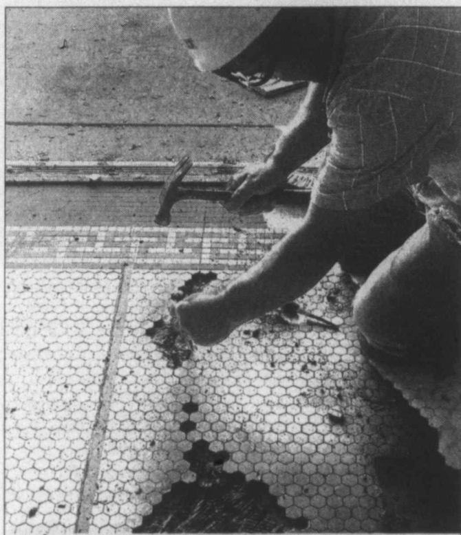
Period floor tiles ... The honeycomb tile flooring, 100 years old, was painstakingly repaired where needed, during the Lynn County Courthouse restoration project. This tile flooring is in the foyer and hallways, and workers were busy last week finishing up the repairs on the floors in time for Saturday's upcoming grand rededication ceremonies at 2 p.m.
