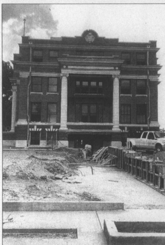
West entry ... Work continues to progress at the Lynn County Courthouse historical restoration project, with soil filled in on the west side of the courthouse. A retaining wall is being built next to a sidewalk for handicap access to the building, from the west entry to the street.
