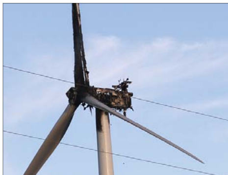
A Vestas V100 wind turbine at the Salt Fork Wind Facility near Jericho was destroyed last Wednesday when a fire burned up the nacelle and one of the turbine blades. Southern Company, which owns the facility, said the cause is under investigation. ENTERPRISE PHOTOS / TOP/JOSH ALLRED, (BOTTOM) ELIANA ESTLACK
