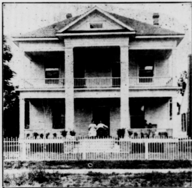
THE NEW METHODIST PARSONAGE JUST FINISHED, AT RICHMOND, TEXAS, BRENNAM DISTRICT, AT A COST OF ABOUT $3300.
