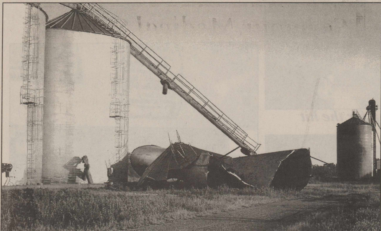
High winds destroyed this grain elevator in Truscott last Wednesday.
