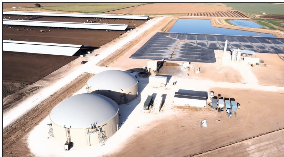
The methane or anaerobic digester harvests methane-rich biogas and fertilizer from the dairy manure, providing another economic revenue for dairies. (Texas A&M AgriLife photo by Juan Piñeiro)
