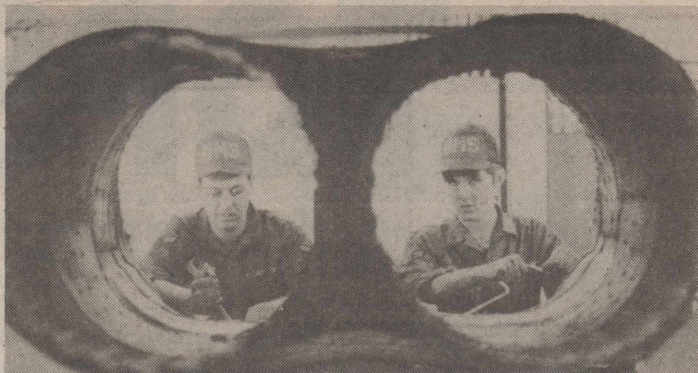
1979 Two OMS members work on a T-38 boattail.
