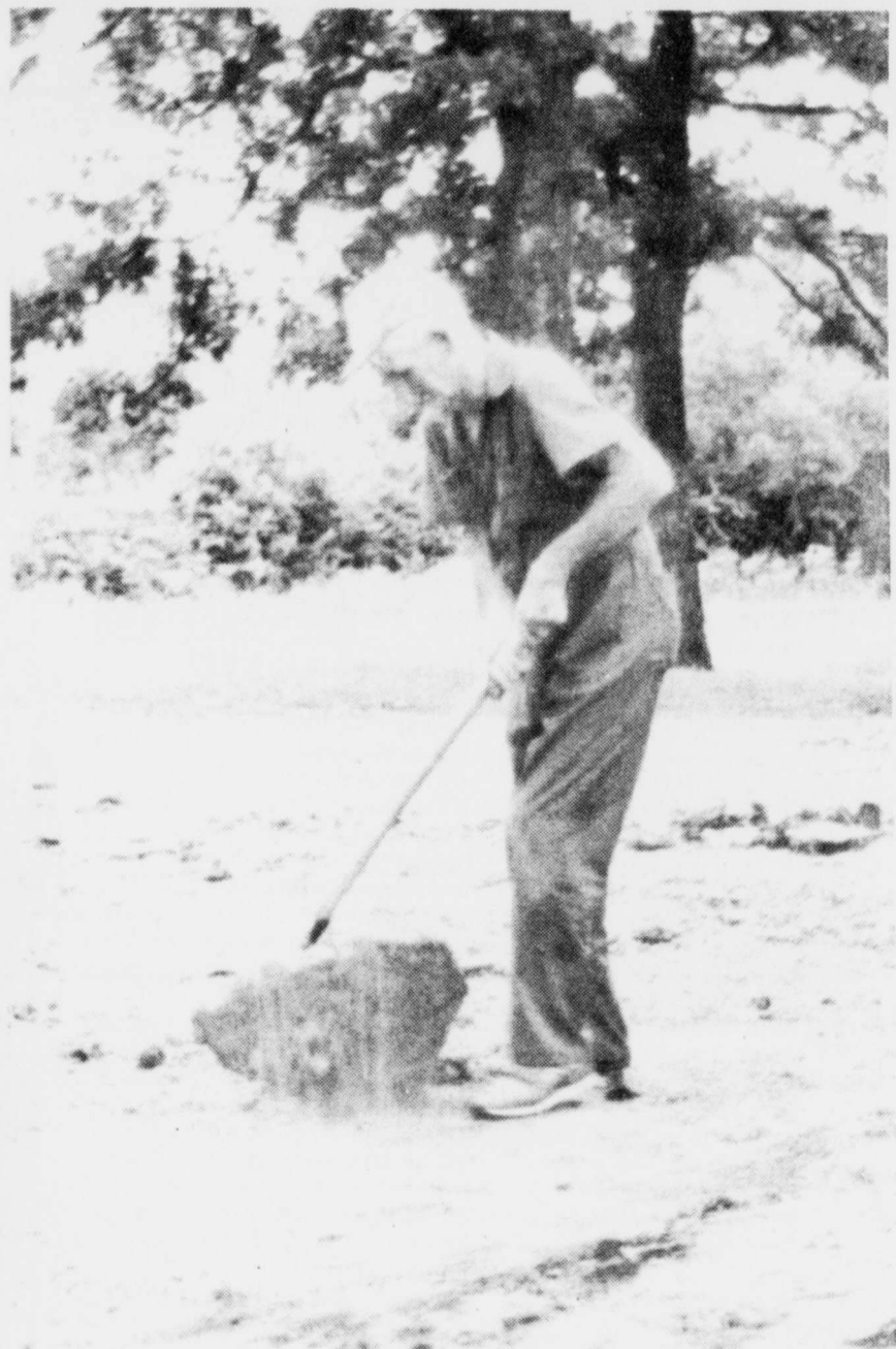
NEW CHURCH! Bro. Gary Orr and Jesse Brown began the groundwork for the new Maple Springs Church this week. Everyone hates to see the old
