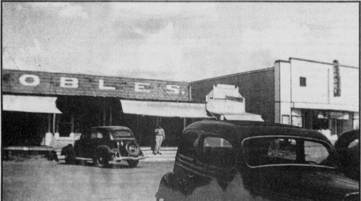
LONG AGO DEPORT-this photograph was brought in by Ed Helleny, who got it from Mac Webb. Taken in the 1940s, it shows Nobles grocery when it was on the east side of main street. Close examination of the tiny building between the two big buildings reveals the sign says "Vogue Beauty Supply". The large building on the right was the Deport theater, which burned in the 1960s. Ed Helleny owned the theater for a number of years.
