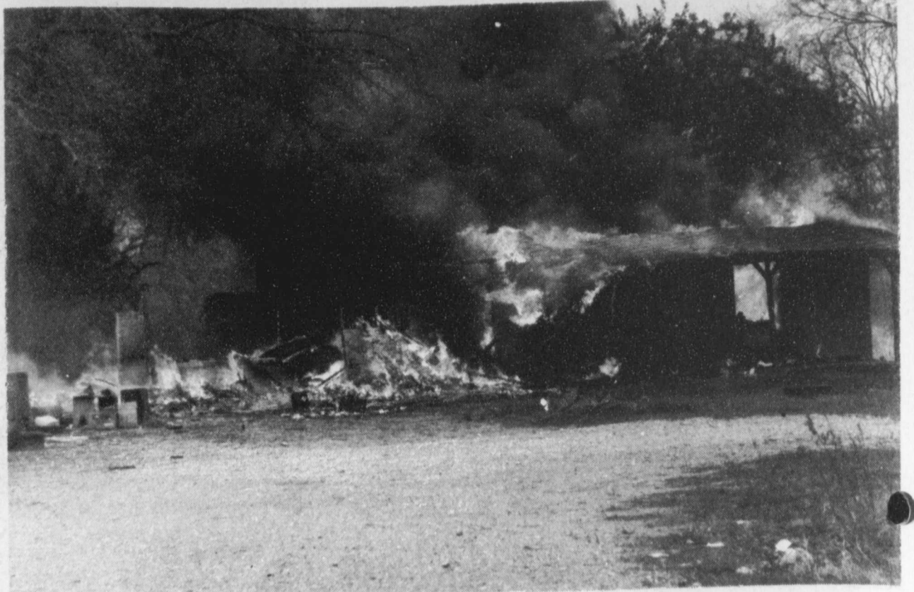
DESTROYED —this house in Cunningham was completely destroyed by fire of an unknown origin Saturday, April 3rd. The empty house belonged to Geneva Norwood and was completely uninsured. Cunningham Volunteer Fire Department responded to the blaze, which was out of control when they arrived. (Staff Photo by Thomas Nichols)
