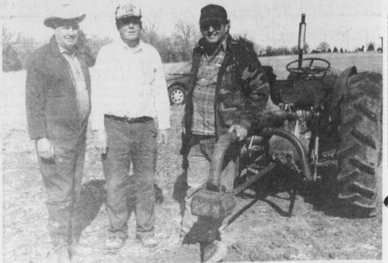
WORKING-volunteers have been busy constructing a tabernacle at Shady Grove Cemetery. From left to right are Stanley O'Brien, J.M. Fisher and Calvin Day. The roof on the structure went up Tuesday Feb. 23. (Staff Photo by Nanalee Nichols)
