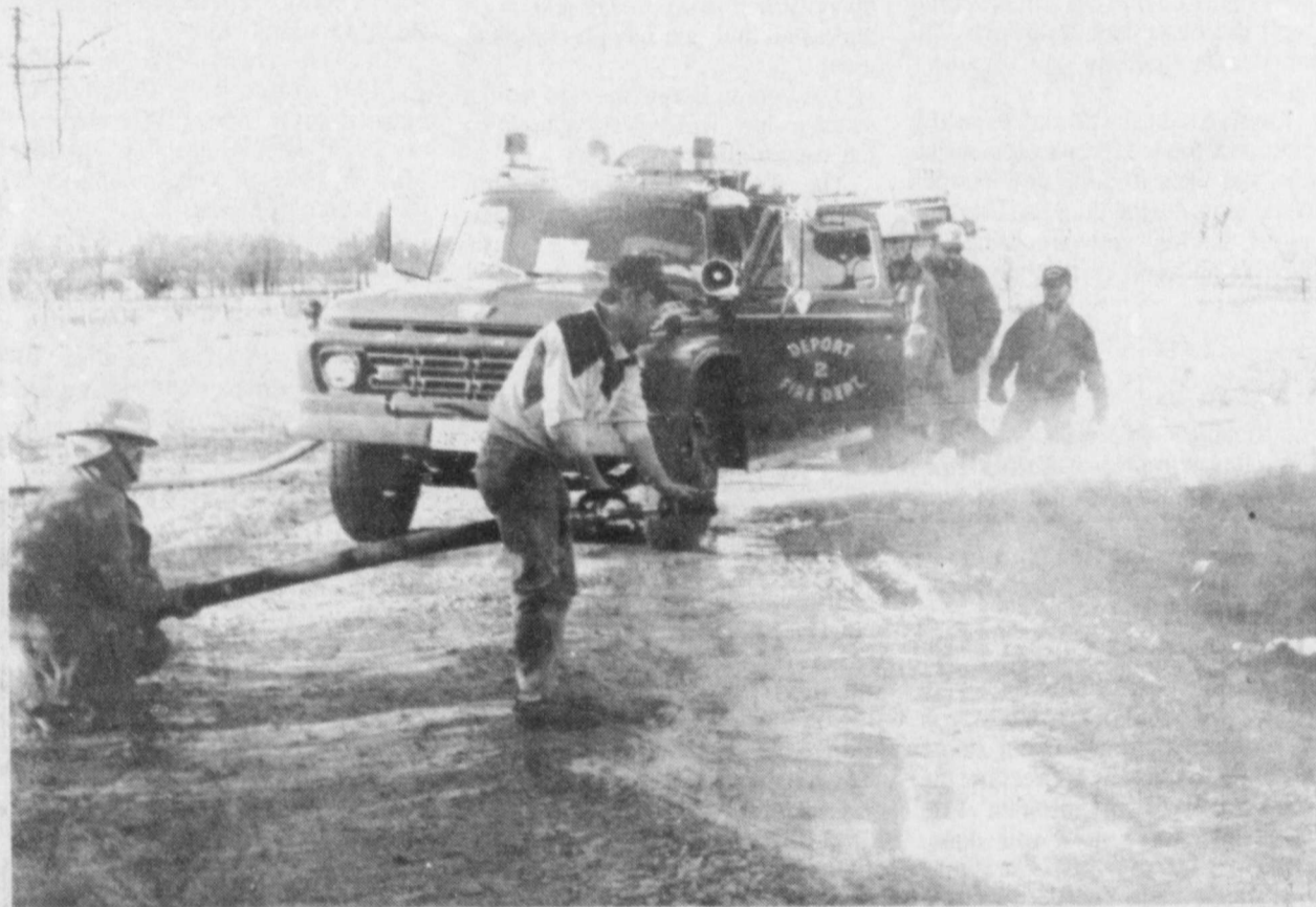
TESTING, TESTING-Deport volunteer firemen tested the new dry fire hydrant installed at the home of Thomas and Nanalee Nichols. The hydrant is located in a pool and will provide nearly instant water in case
