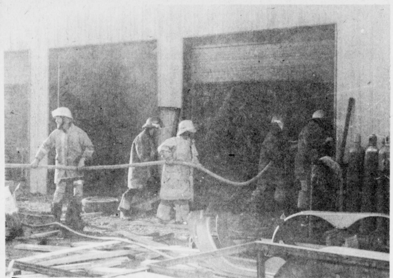
HEAVY DAMAGE -Armadillo Trailer Manufacturing sustained severe damage to the structure Tuesday afternoon as fire roared through the building. Deport Volunteer Firemen extinguished the fire, which
