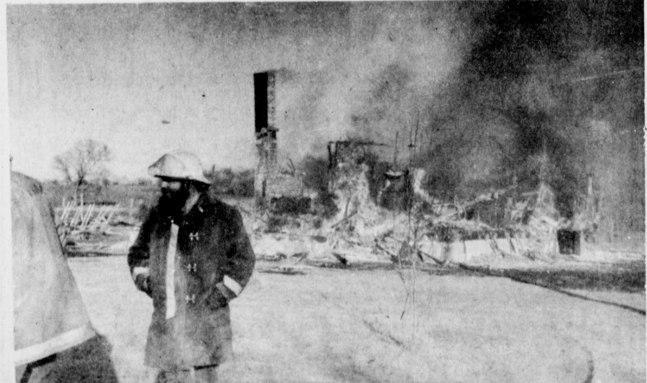
DESTROYED -the home of Rhett and Sherry Clarkson and their three children was totally destroyed by fire
